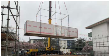
THE NEW-LOOK STANLEY, WITH (TOP LEFT) AN ARTIST'S RENDITION OF THE JUNIPER, AND (BELOW) PRE-FABRICATED MODULAR HOUSING BEING CRANED INTO PLACE.
